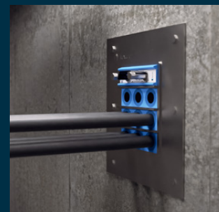
Partition wall between two areas
